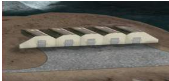
Rocket Motor Storage Facility (under construction)
