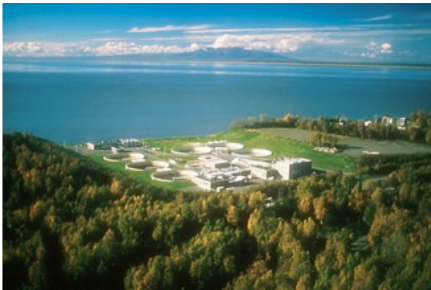
The John Asplund Wastewater Treatment Plant was named best service provider in a national competition.
