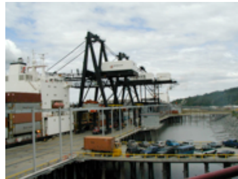
Existing cranes at Port of Anchorage
