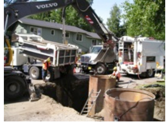
AWWU crews use large round steel tubes to protect workers repairing a utility break
