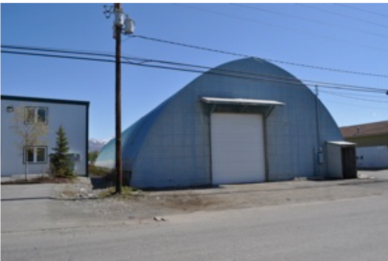
Buildings like this in industrial zones can be redeveloped
