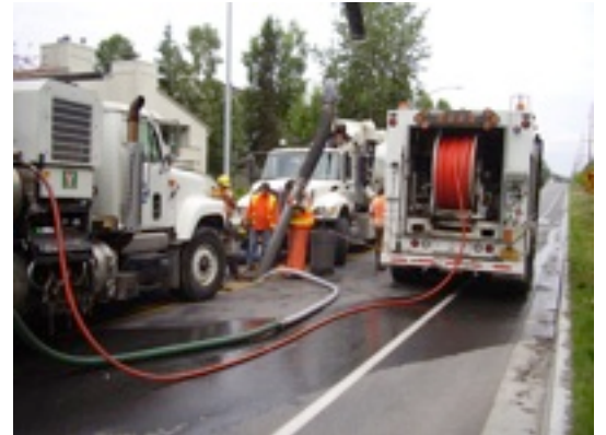
Each year AWWU crews inspect and eliminate plugs in more than 750 miles of
