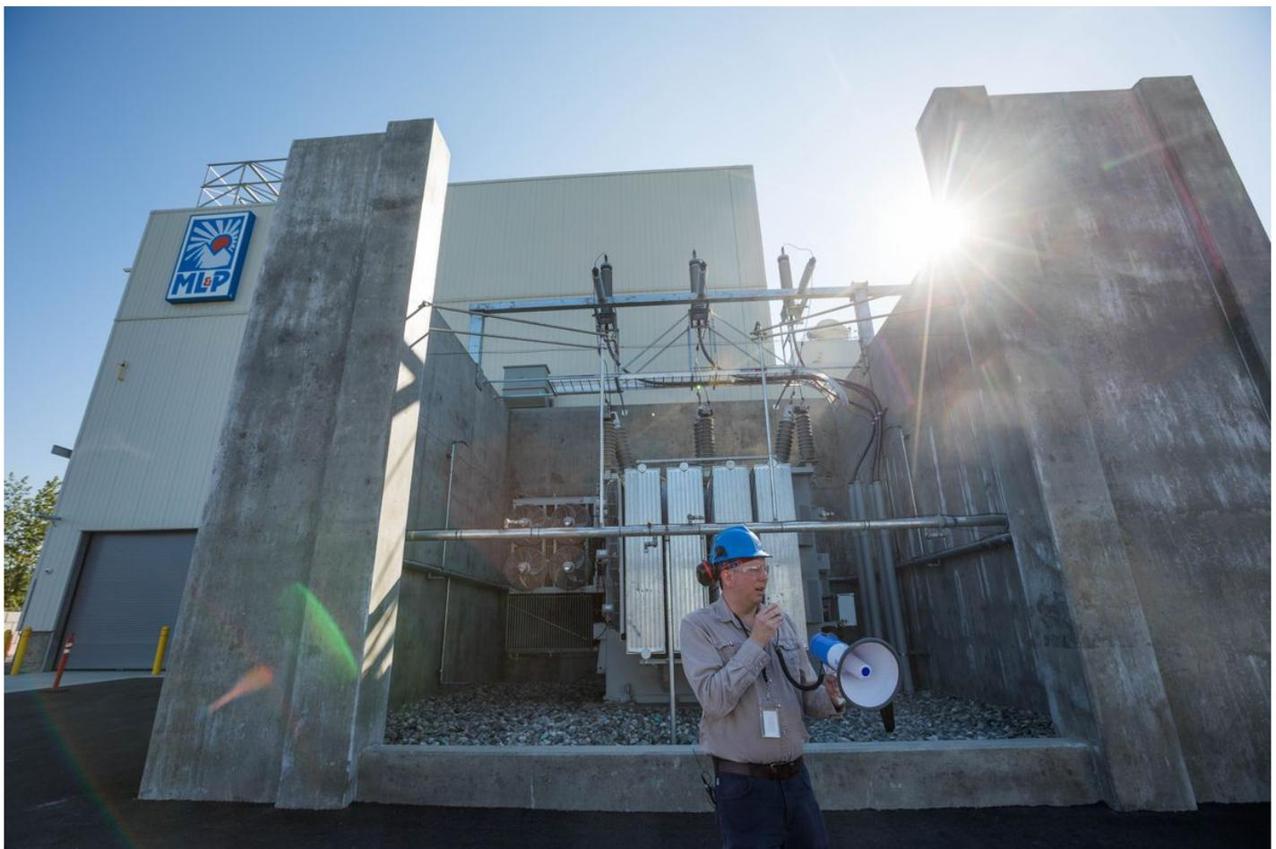
*Plant superintendent Nat Lewis leads a media tour of the George M. Sullivan Plant 2A electrical generation station on July 6. Behind Lewis is a transformer that takes a 13,000-volt current and turns it into a more transmission-friendly 115,000 volts. Plant 2A is Municipal Light and Power's newest power plant, and it generates 120 megawatts through the burning of natural gas. (Loren Holmes / ADN)*
