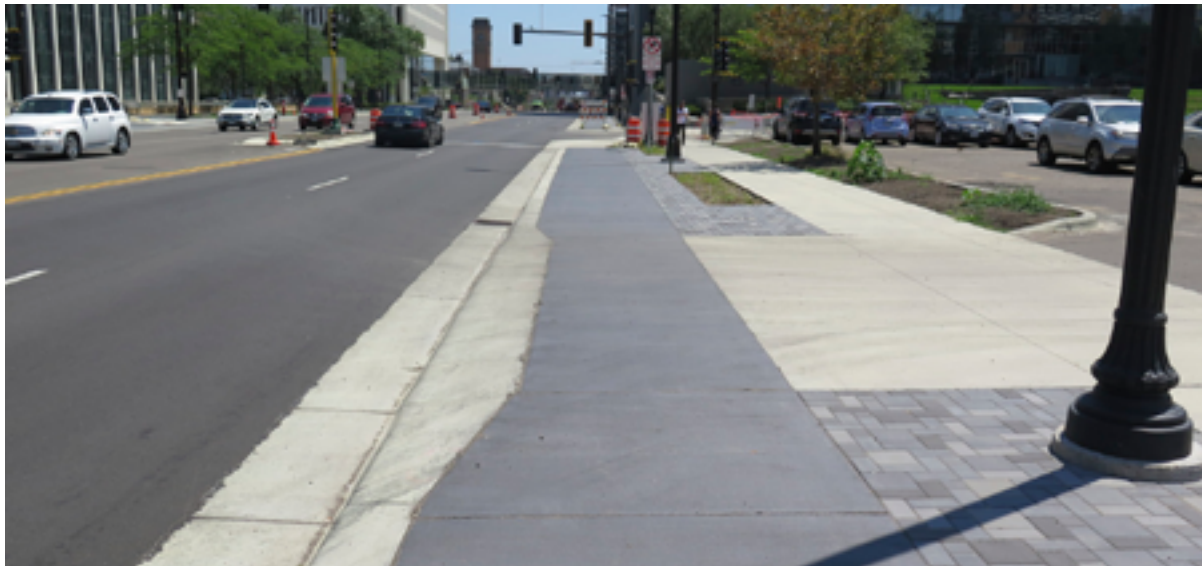
Example of a driveway maintained at-grade with a vehicle apron to manage grade change on the street-side of the separated bike lane.
